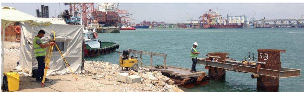
Figure 7. Lateral Load Test Set-up
